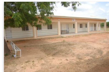
Figure 3: A set of classrooms built for CMin Katsina
