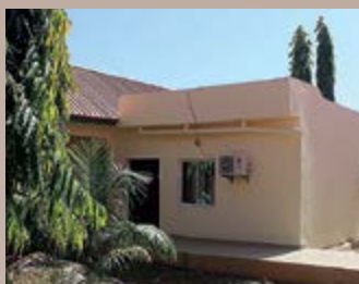
Newly built office at a Health Training Institution
